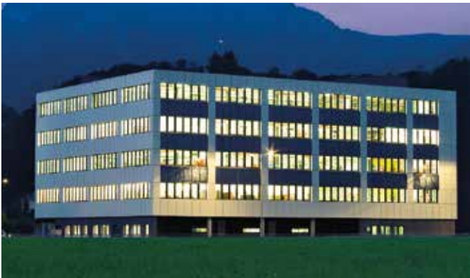
Leister Technologies AG, factory, Sarnen, Switzerland
