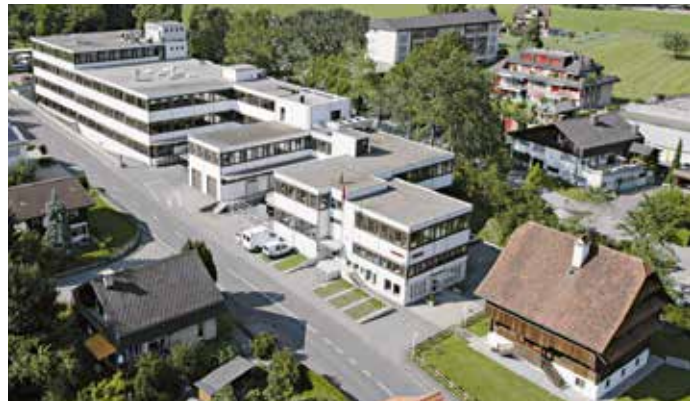
Leister Technologies AG, factory, Kaegiswil, Switzerland
